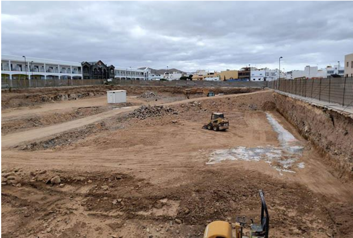
Works in El Cotillo, last October. Photo: I. Leis.
